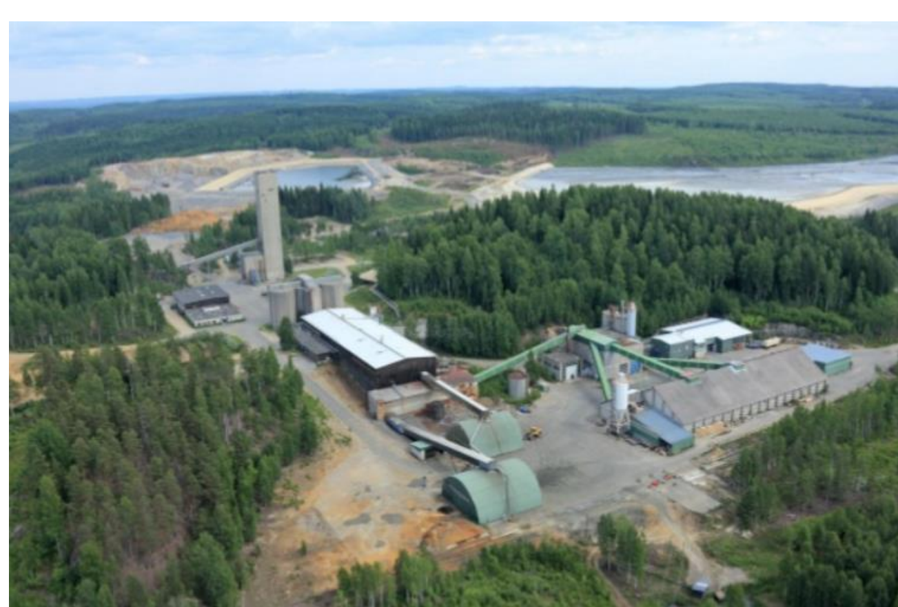
Luikonlahti Cu-Zn-Au processing facility (Finland)
